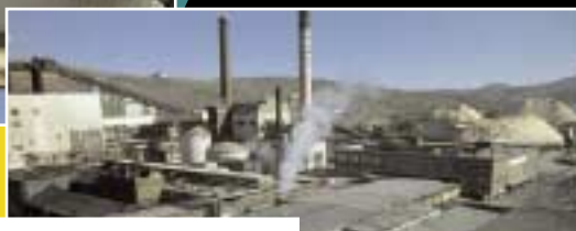
Tembec Inc., Temiscaming, PQ.. Contractor Les Industries Pard Inc.. Over 7000 squares of modifiedPLUS ™ on pulp and paper mill roof since 1985.
