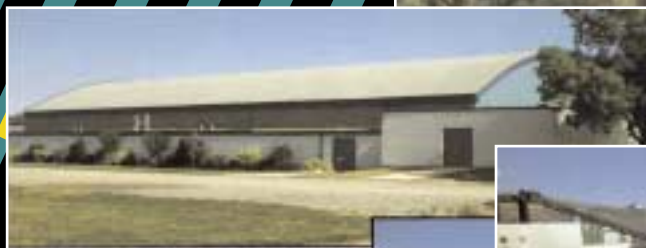
Virgil Centennial Arena, Niagara-on-the-Lake, ON. Contractor Provincial Industrial Roofing & Sheet Metal Co.
