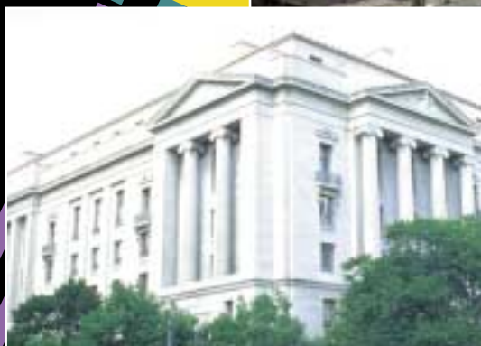
Justice Building - Washington, D.C. Two-ply protected membrane modifiedPLUS ™ system. Contractor Marangos Construction Corp.
